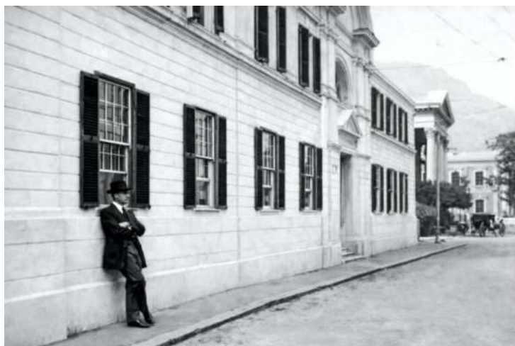
Old Supreme Court Building
