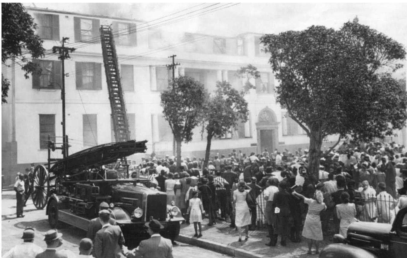
The Fire - Damage to the front of the building (Photo: Cape Times)
